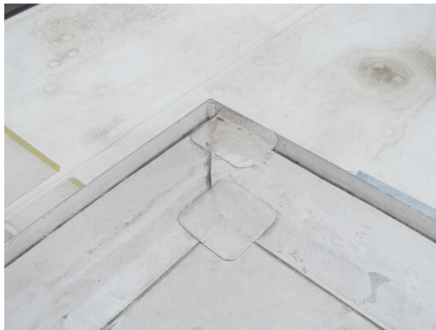
Roof system perimeter termination
