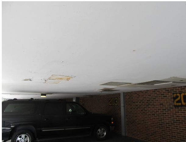
Previous repairs at soffit
