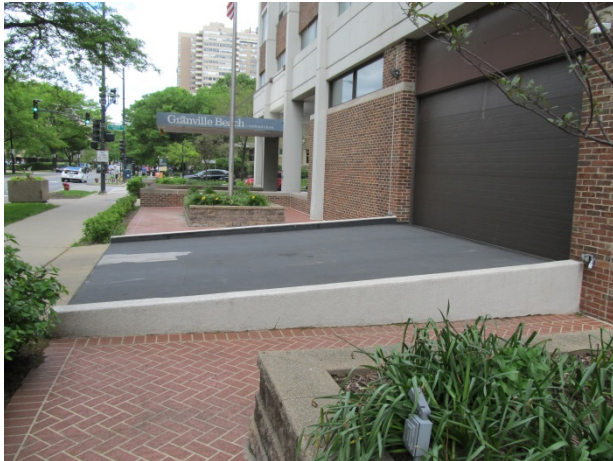
Vaulted systems at west perimeter
