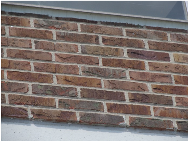
Tower masonry joint condition
