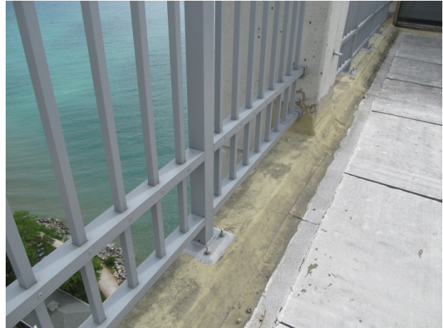
Railing at mount
