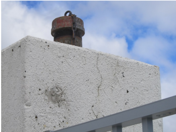
Concrete crack
