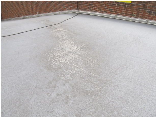
Traffic coating west at 2 nd floor
