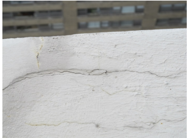
Concrete crack
