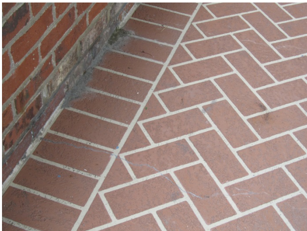
Cracks in concrete/coating at west perimeter
