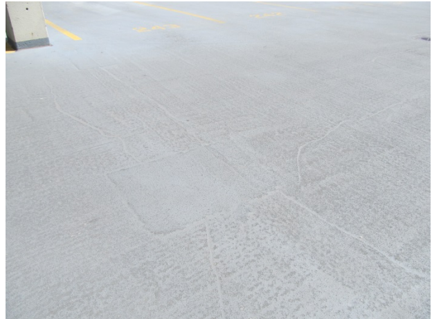
Traffic coating west at 2 nd floor
