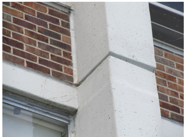
Previous concrete repairs
