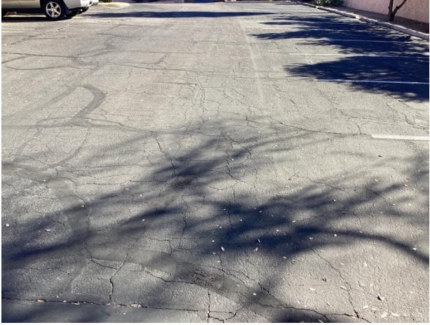
Extensive pavement cracks
