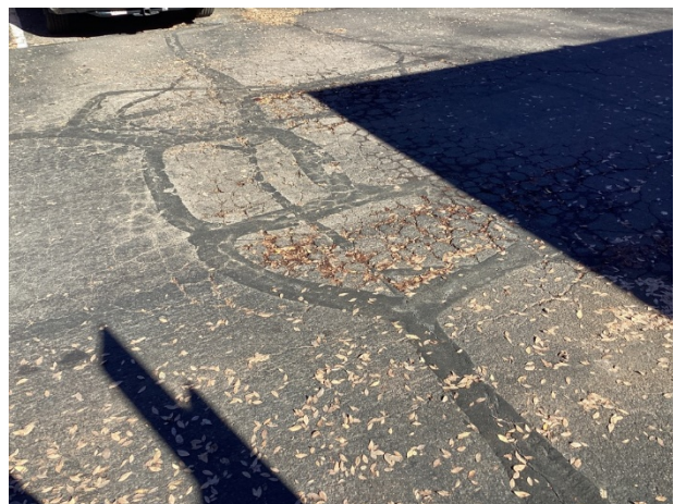
Significant alligator cracks
