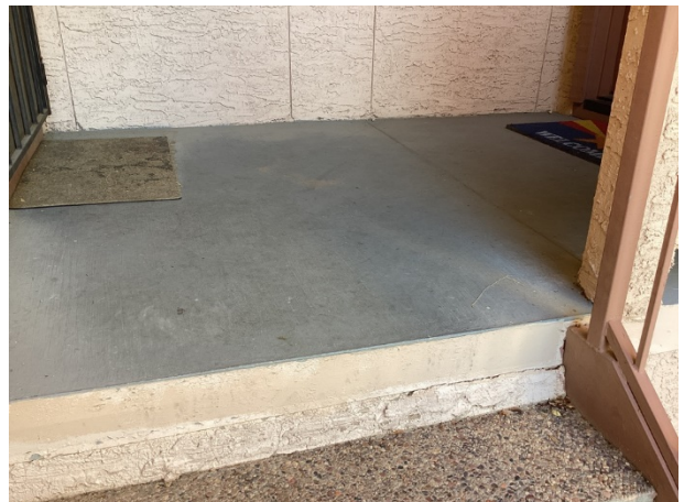
Concrete topping with coating
