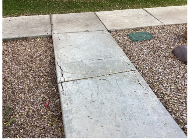
Sidewalk cracks
