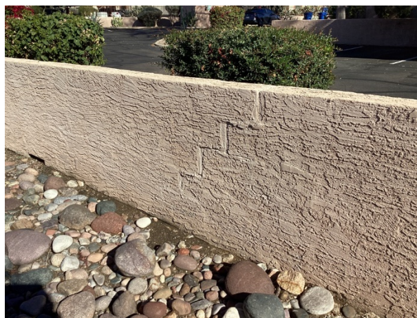
Step crack at west perimeter wall
