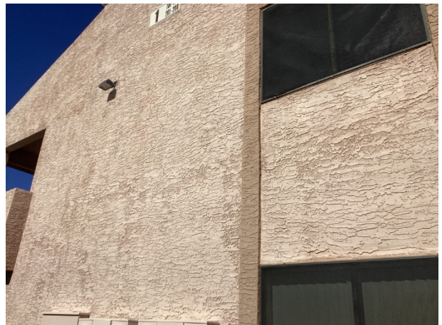
General fade at south facing elevation
