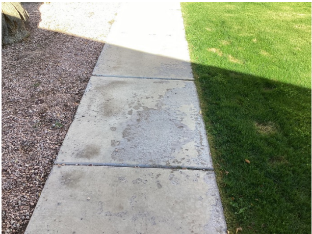
Sidewalk spalls
