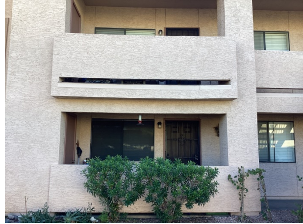
Possible deflection at Building 5, note this location has carpet present
