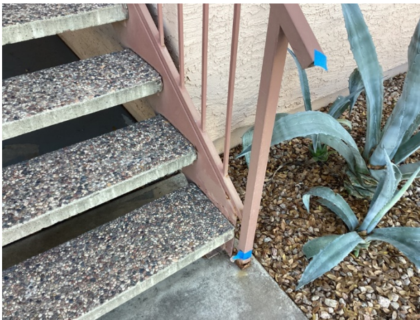
Corrosion at Building 8
