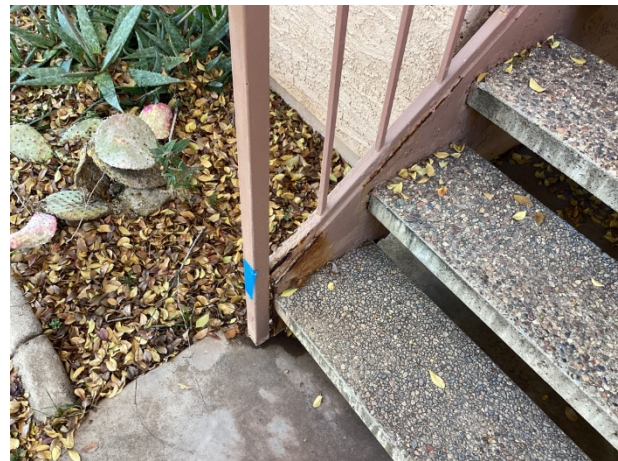
Significant corrosion at Building 5
