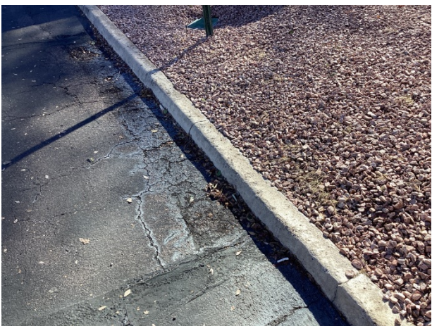
Concrete curb spalls
