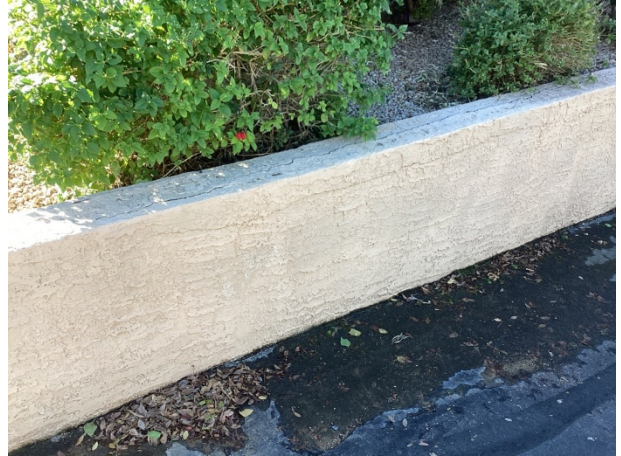
Stucco cracks at retaining wall by Building 6
