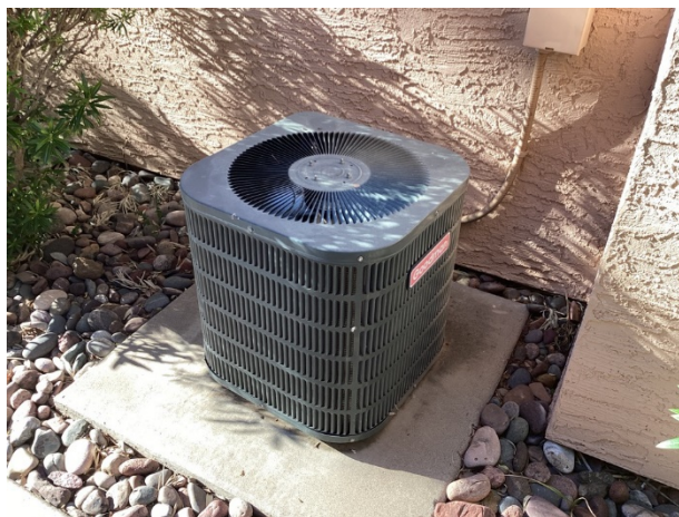
Split system condensing unit
