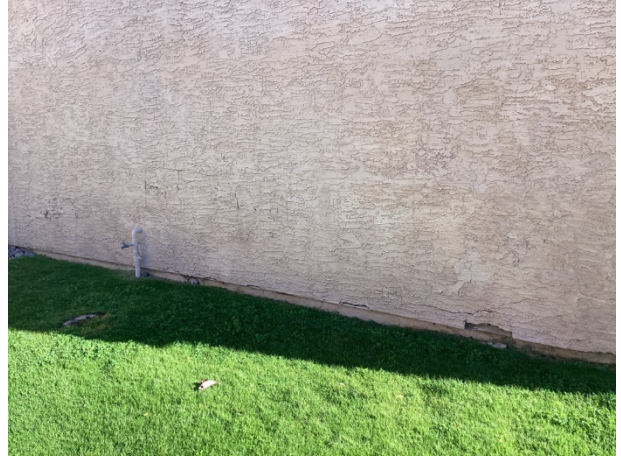
Stucco cracks and peeling paint at cabana
