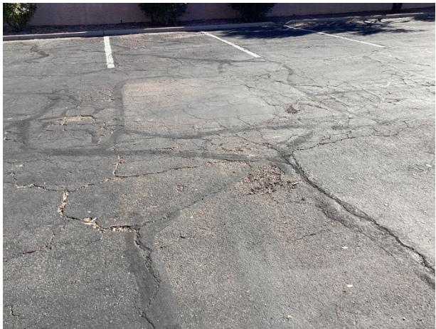
Alligator cracks and potholes
