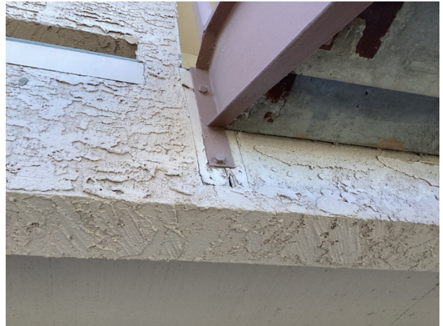
Deterioration at fastener
