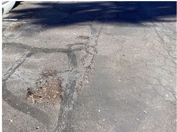
Pavement pothole formation
