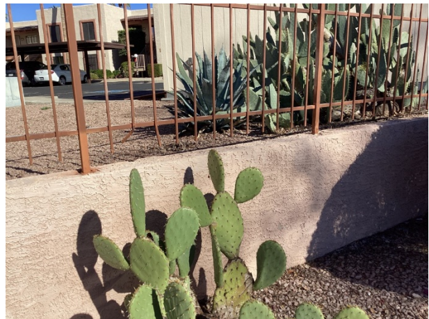
Wall paint finish deterioration and damaged fence pickets
