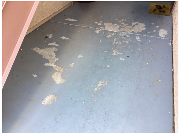
Coating delamination at unit entrances
