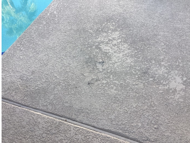
Textured coating delamination
